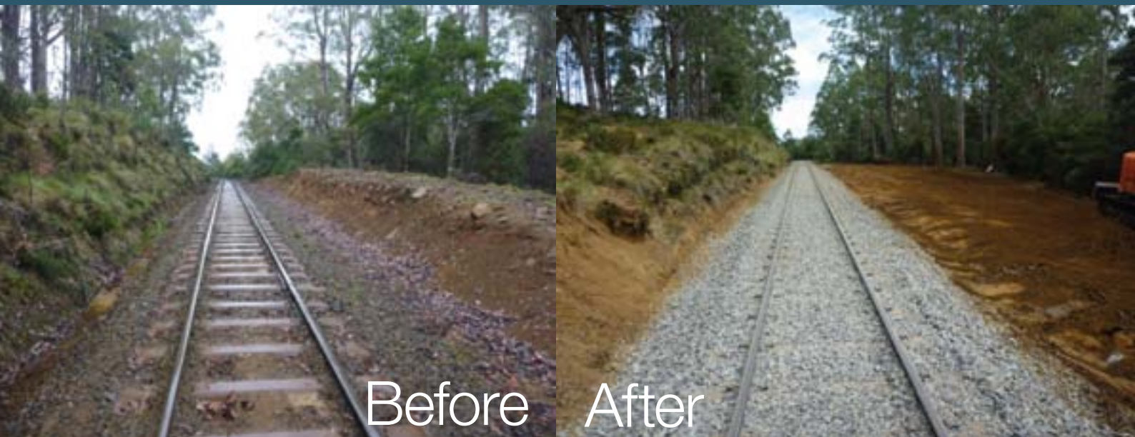
Pictured above before and after the formation works.
